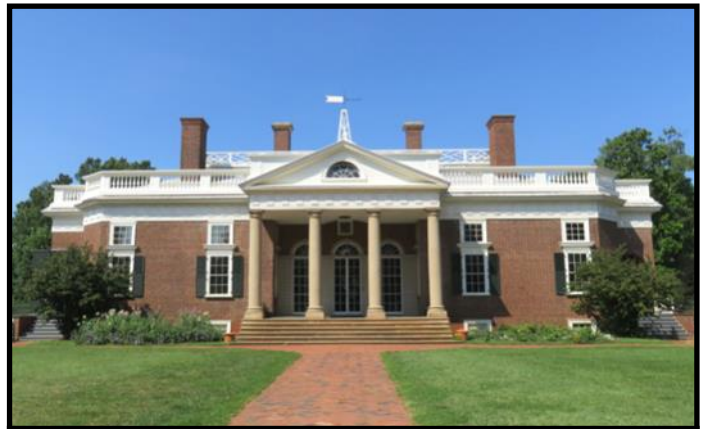
The East Front of Monticello which faces the gardens and valley
