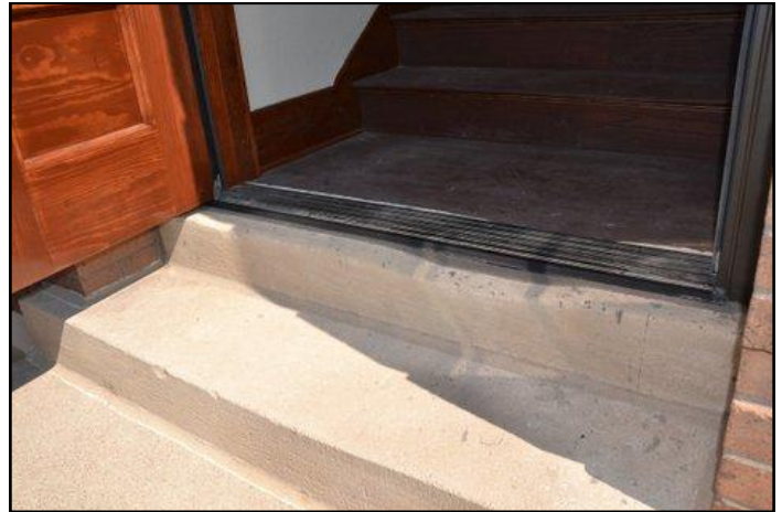
TIRED STEP —This concrete staircase was worn down by patients going to see Bill's father, 'Doc' Wilcox.
