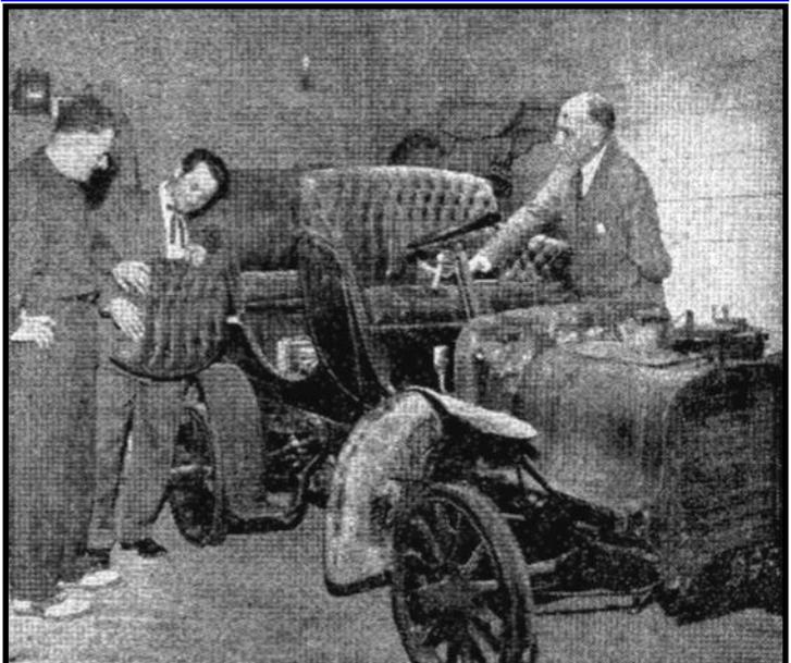
Gatewood, left, Brill, center, and L. M. von Schilling inspect progress of restoring Brill's 1906 one-cylinder Cadillac, with double tulip body.
